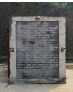
FAR LEFT: Brick wall without fibre reinforced polymer (FRP).
