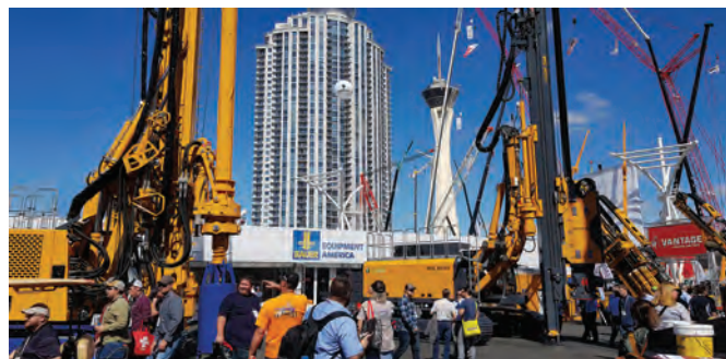
Bauer displayed its drilling rigs as well as products from its subsidiaries Klemm and RTG, plus Bauer MAT Slurry Handling Systems plant.
