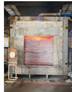
FAR LEFT: Actual installation of blast resistant roller shutter.
