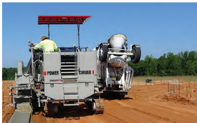
Power Curber 5700-D curb and gutter machine.
